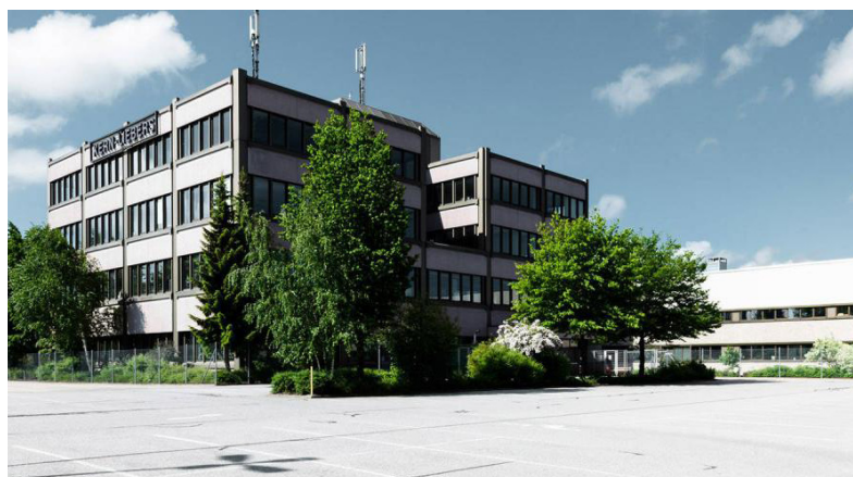
Fig. 3: Checkmk's main site is located at the company's headquarters in Schramberg
